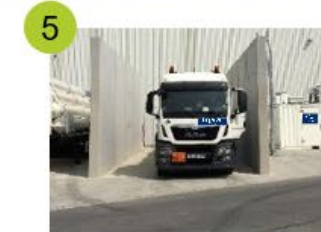
Hydrogen filling station
