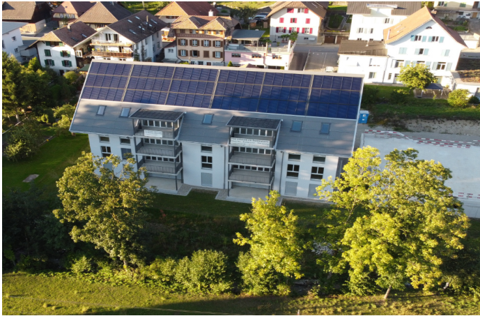
The apartment building in Huttwil, built in 2020, is covered with 160 m 2 of solar collectors. These provide enough space heating and hot water to supply the eight apartments all year round. Photo: Jenni Energietechnik AG
