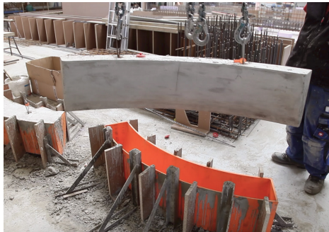
On-site casted window arc concrete part
